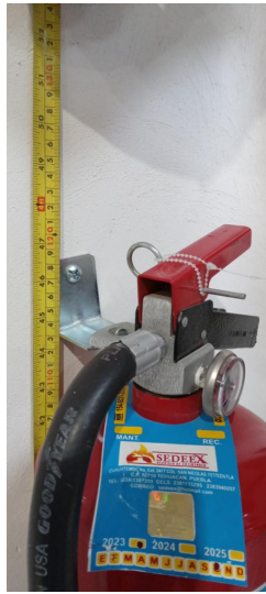
Fire extinguisher installed within the height set by the law.jpg
